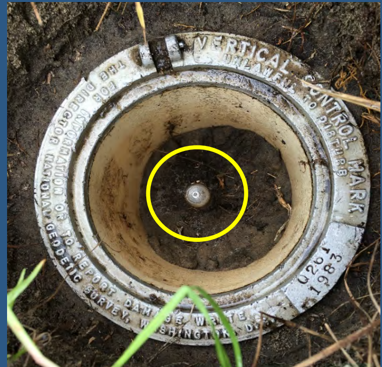
Access Cover Open
